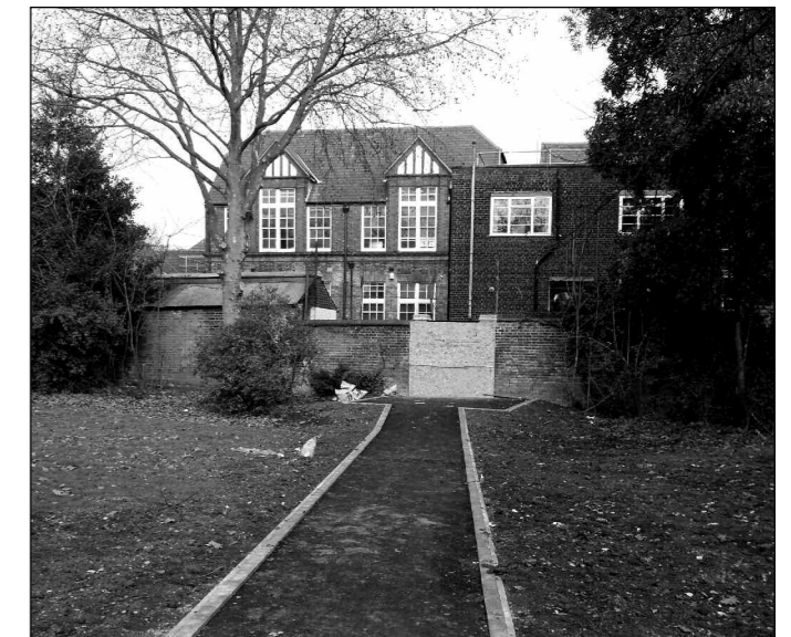
A new path, under construction from Downhills School through to Downhills Park
